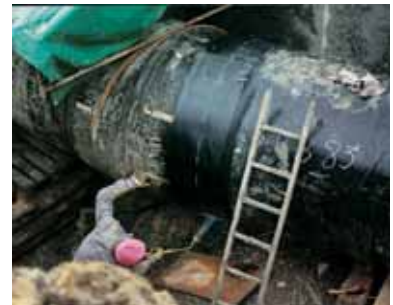
WPC-C50 installation on big pipe Our range of 2-layer mastic coated sleeves balance performance, economy and ease of installation. No primer required, simple tools as hand or power brush, propane torches, etc.
