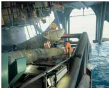
WPC100M in offshore application The combination of a one piece sleeve (unisleeve) and fast shrink response allows rapid and reliable installation under lay barge conditions, with or without joint in fill systems.
