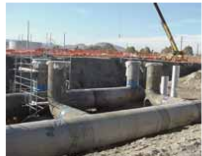
WATERWRAP on large diameter water pipes Special formulated low preheat adhesive makes WATERWRAP suitable for internal welding application under approved conditions.
