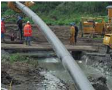
DIRAX application for river crossing The special glassfiber reinforced sleeve gives the material a high abrasion resistance while remaining flexible to follow bending radius.
